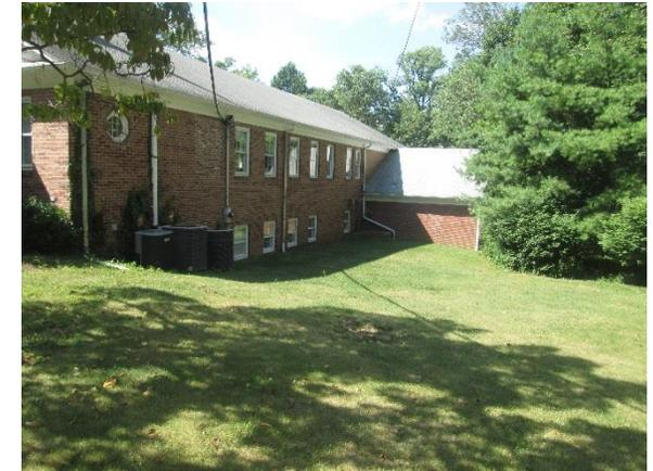
Parking spots adjacent to the building and in the northwest section of the parking lot can be replaced with porous asphalt to capture and infiltrate stormwater. Downspouts on the east side of the building can be disconnected and redirected into a rain garden to capture, treat, and infiltrate roof runoff. A preliminary soil assessment suggests that more soil testing would be required before determining the soil's suitability for green infrastructure.
