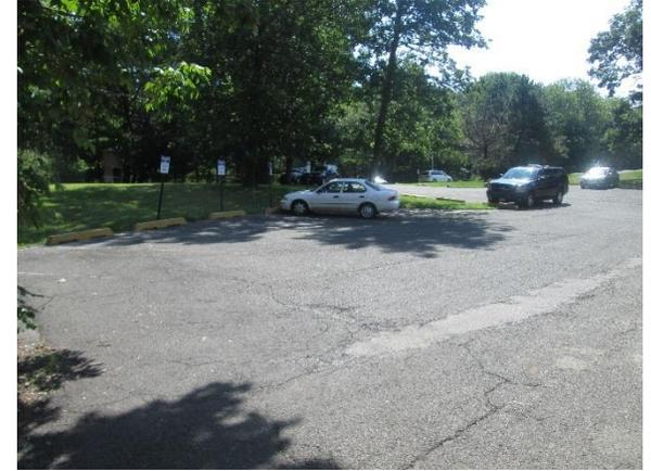
Parking spaces can be replaced with porous asphalt to capture and infiltrate stormwater runoff. A preliminary soil assessment suggests that more soil testing would be required before determining the soil's suitability for green infrastructure.
