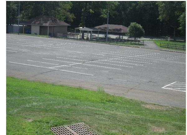
Parking spots south of the school can be replaced with porous asphalt to capture and infiltrate stormwater. A preliminary soil assessment suggests that more soil testing would be required before determining the soil's suitability for green infrastructure.
