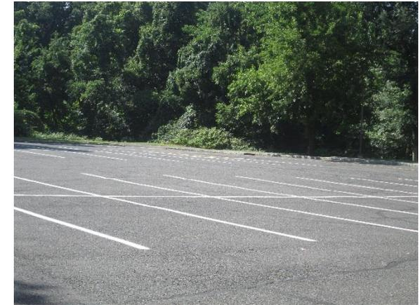
Multiple rows of parking spaces west of the school can be replaced with porous asphalt to capture and infiltrate stormwater. A preliminary soil assessment suggests that the soils have suitable drainage characteristics for green infrastructure.
